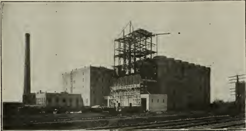
1,000,000-bushel fireproof Grain Elevator, constructed of Hollow Tile Building Blocks, for Albert Schwill & Company, South Chicago.
